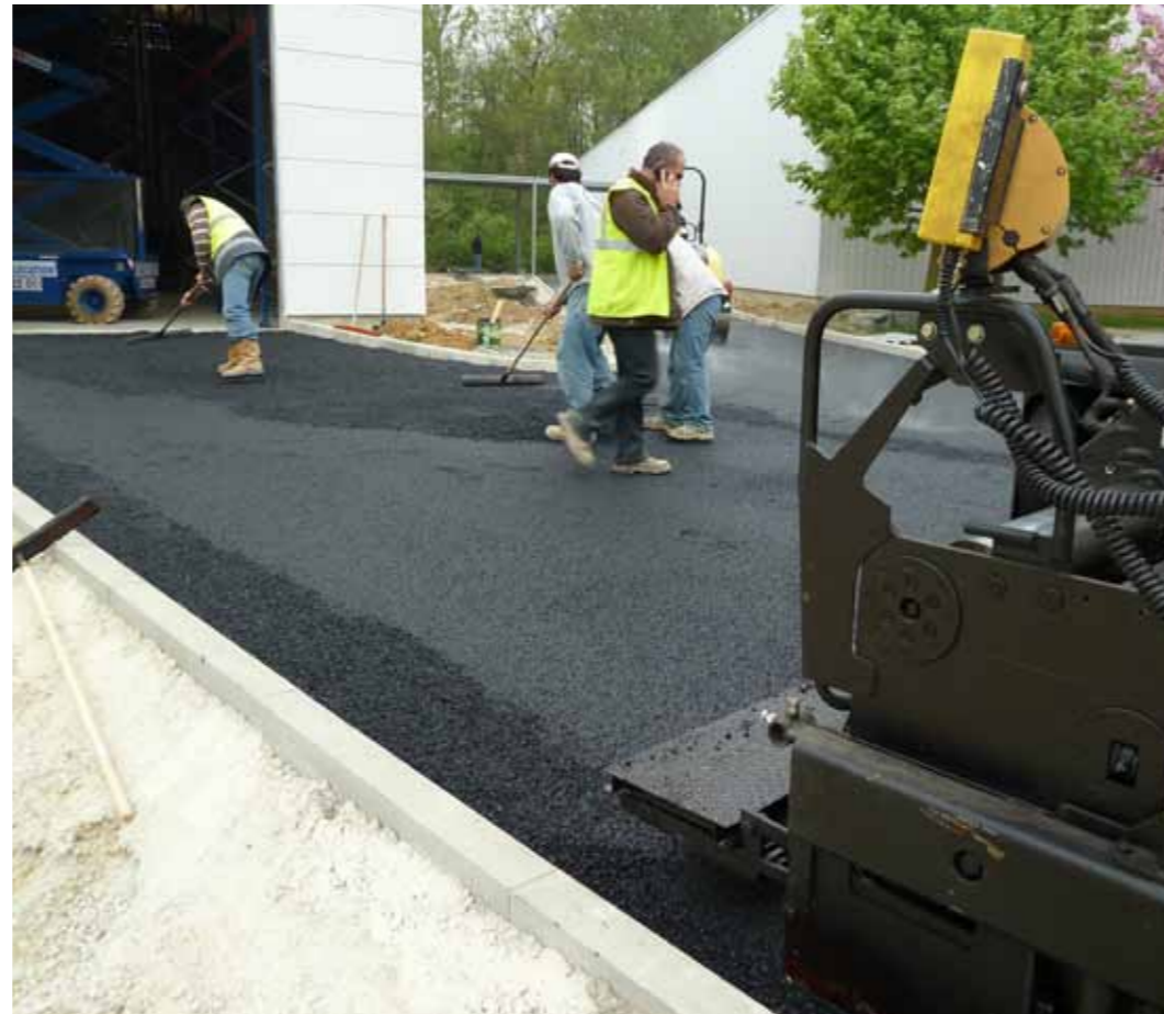
^ The pavers work well when placing asphalt for a new warehouse.
